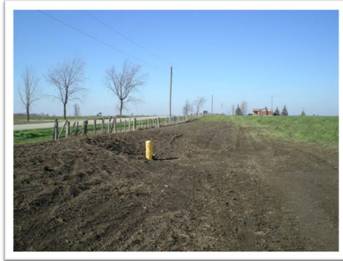
A water and sediment control basin constructed to keep soil on the field
