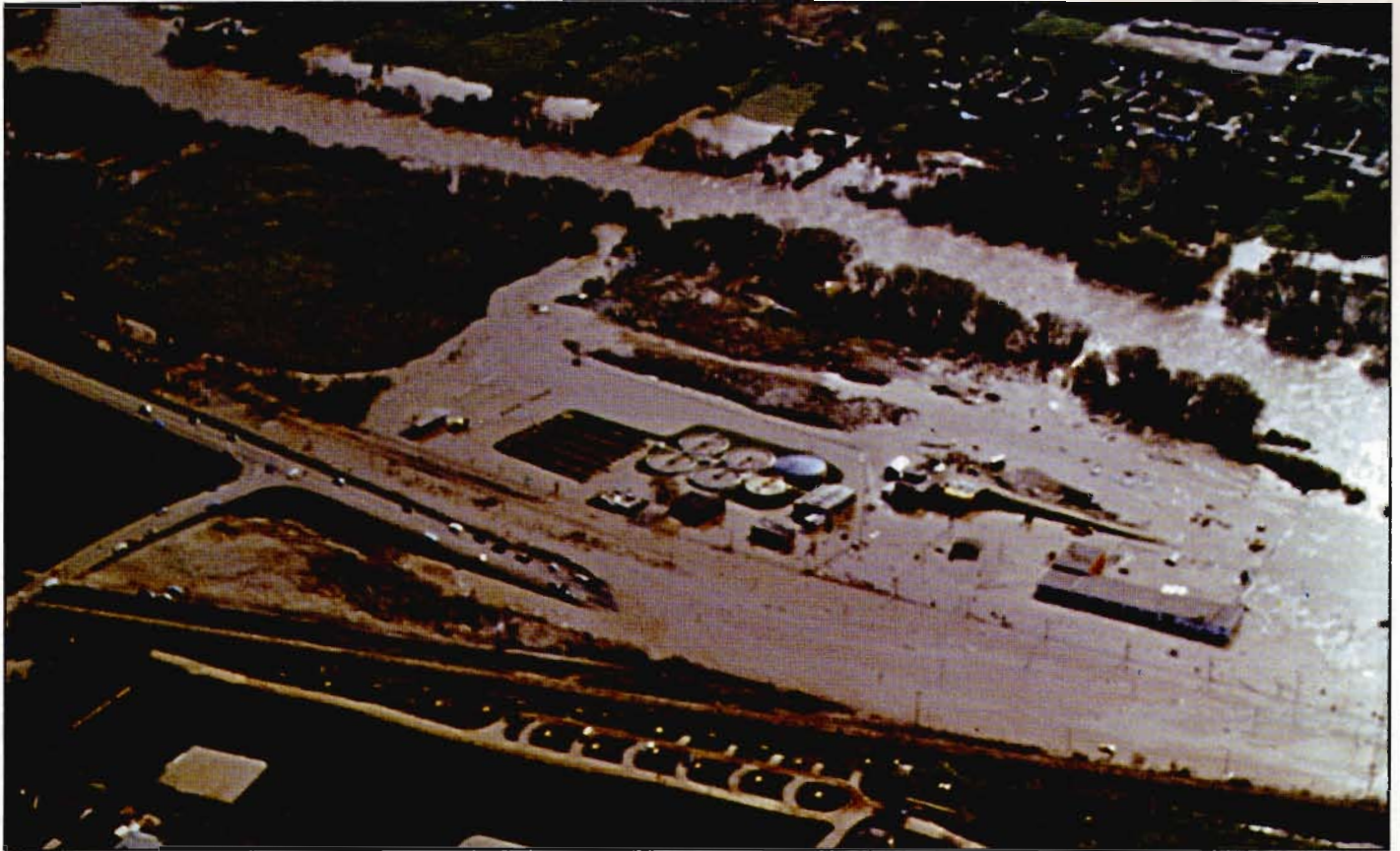
Galt, South - Highway 24 closed- Sewage Plant West 5:30 p.m. May 17, 1974
