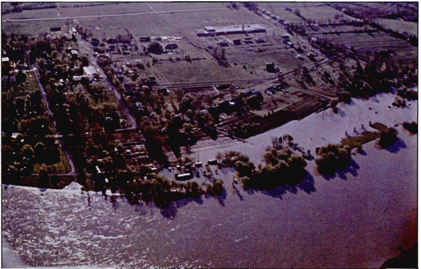
Cayuga - Flooded Houses on Inside Bend North 8:00 a.m. May 18, 1974
