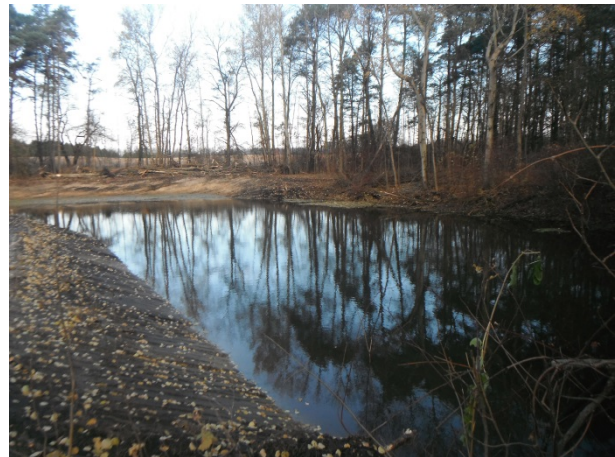
Figure 12: John Kertez's pond after, Entire pond, 50ft expansion of the North side (near the top of photo).
