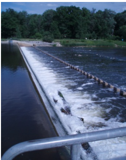
Mannheim intake, Grand River
