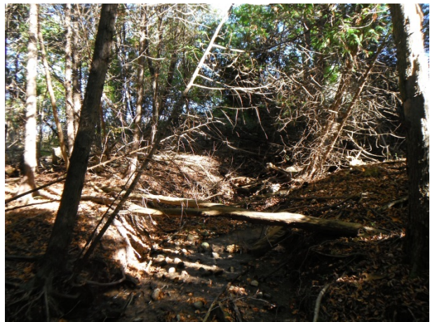
Figure 28: Mr. Vamos' pond outlet downstream of East arm.
