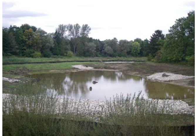
After: One of the off-line ponds constructed in 2009.
