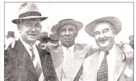
Photos from top: sod turning ceremony for the Shand Dam; construction in October 1940; a visit to the worksite; logs on GRCC truck; mayors from the three communities that benefited from the dam were William Pelz of Preston, Joe Meinzing of Kitchener and J. P. Ryan of Brantford.
