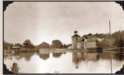
The Harris Woolen Mill in the 1890s, shortly after it was rebuilt of stone.
